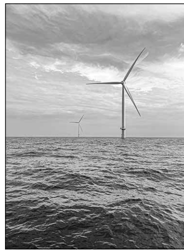
Two wind turbines, in Federal waters, 27 miles off Virginia Beach, part of the Coastal Virginia Offshore Wind project. Photo by U.S. Bureau of Ocean Energy Management.
