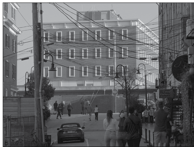
Basking in rare sunshine, the McIntyre Building looms over Ceres Street. On Tuesday, the bidding in the GSA's online auction had risen to $8.5 million, putting the parcel beyond our reach. This is most unfortunate. If we were to redevelop this property, our first priority would have been to put the Post Office back where it belongs. We'll have to settle for Plan B. Whosoever does acquire and redevelop this property, beware; fail to bring back the Post Office, and you will face our eternal opprobrium.
